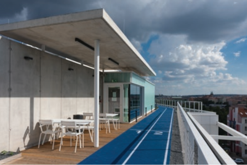
Visionary office building, Prague
