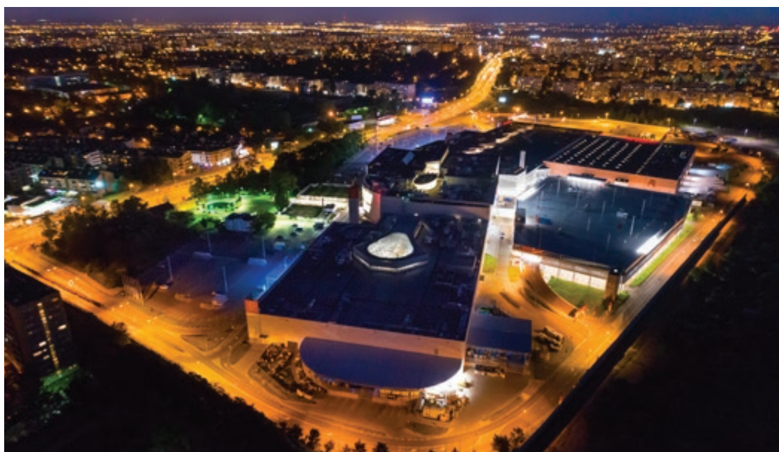
Centrum Handlowe Wola Park (rozbudowa), Warszawa Wola Park shopping centre (expansion), Warsaw
